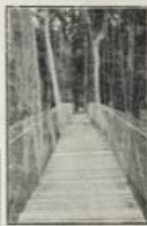
Suspension Bridge 100 Feet Long, 100 Feet High. For use of Footpaths.
